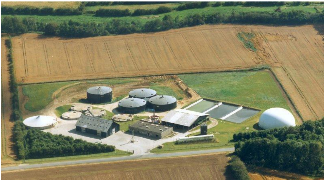
Figure 1.7. Anaerobic digestion plant
