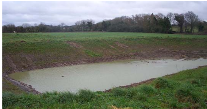
Figure 18: Grange earth-banked tank after emptying (2001)
